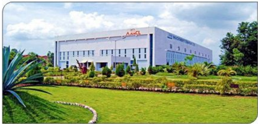
Works at Nagpur
